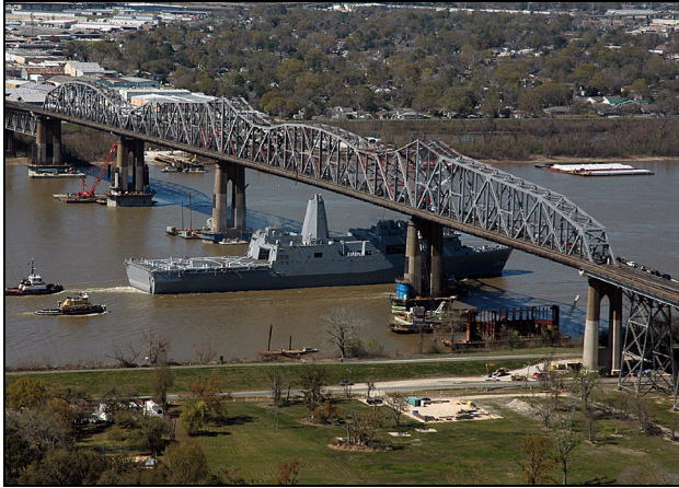
Huey P. Long Bridge, roadway portion on far side of the bridge. Note: the simple span truss on the left was also constructed by cantilever methods.
