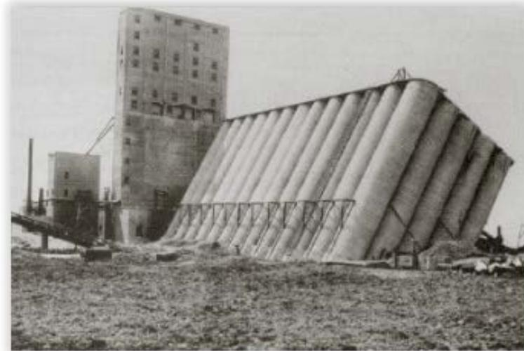
Bearing failure of a silo in Manitoba, Canada (1913)
