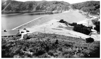
The 110 ft. high state approved, earthen dam with reinforced concrete facing, provides up to 25,000 acre-feet of storage <u>during years of sufficient rainfall.</u> Howells & Howells\* in 1925 had estimated the average annual yield from the
