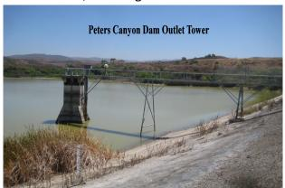
capacity. It's purpose is to regulate the draft from Santiago Dam (Irvine Lake) to lower reservoirs. Distribution to southerly Irvine Ranch was via underground pipeline for one mile to the "High Line Canal". The open channel then carried the flow by gravity several miles easterly across the ranch.
