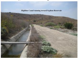
gunite canal lining remain structurally sound today. A "splitter" on the canal just ahead of Siphon Reservoir allowed diversion of water
