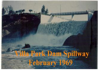
Uncontrolled spillway discharge had peaked at 4,500 cubic feet per second. For several days the
