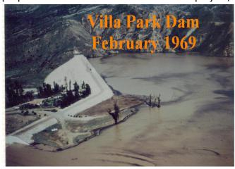
it is kept empty to debris pool elevation except during flood operations. In February of 1969 a combination of extreme rainfall events produced a volume of inflow exceeding design engineers estimates. After the upper dam (Santiago) filled to capacity, Villa Park also filled.
