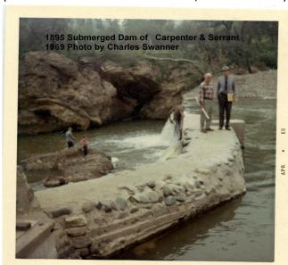
The Carpenter and Serrano "submerged dam" became visible in 1969 when scoured by flood flows released from Villa Park Dam. A photo (below left) of Carpenter and Serrano's dam was taken in the following spring by long-time Santa Ana attorney and historian Charles Swanner.
